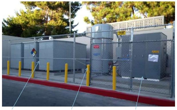
Reactors, Instrumentation and other devices under test Cryostat – Superconductor Unit Cryogenics – Cooling system
